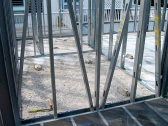
CONCRETE FLOOR SLAB EMBEDS STUDS AS TORSION RESISTANT DIAPHRAGM
