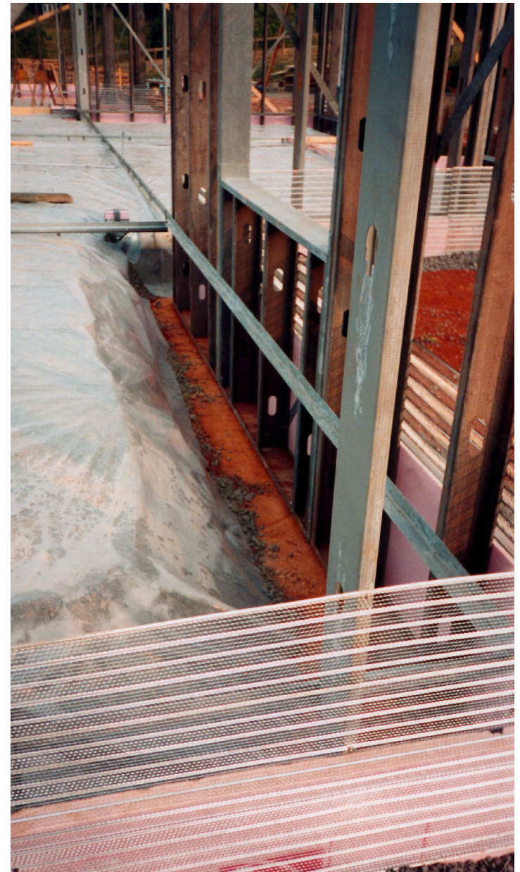
Pin prefabricated wall panels to concrete footing
