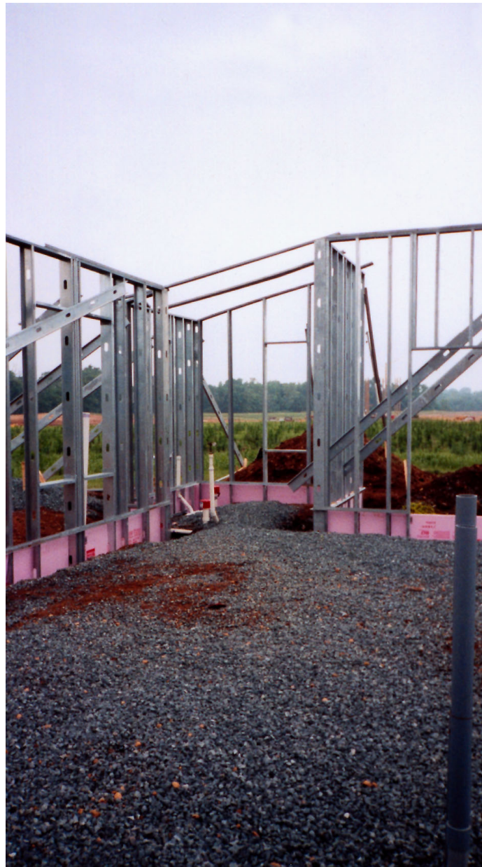
Pin prefabricated wall panels to concrete footing
